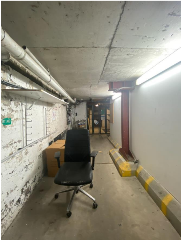
Figure 13: View of lower ground floor level
