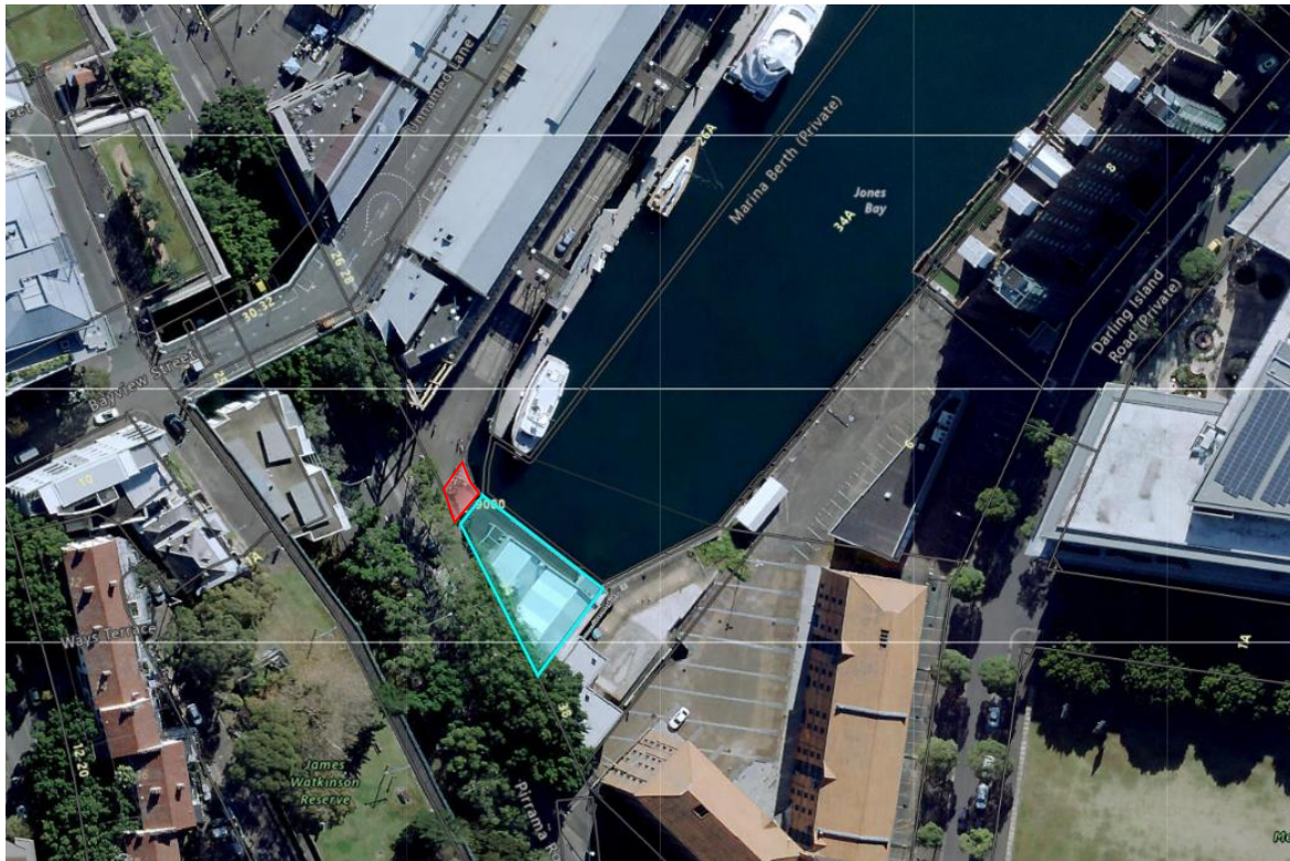
Figure 1: Aerial view of the site and surrounds. Subject site shaded in blue and red, with the portion in red being located on the adjoining site at 26-28 Pirrama Road.
