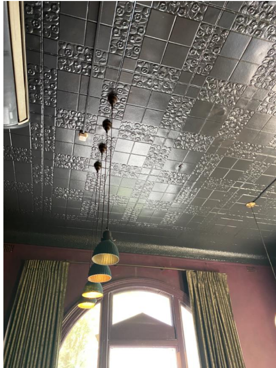
Figure 8: View of ground floor level ceiling
